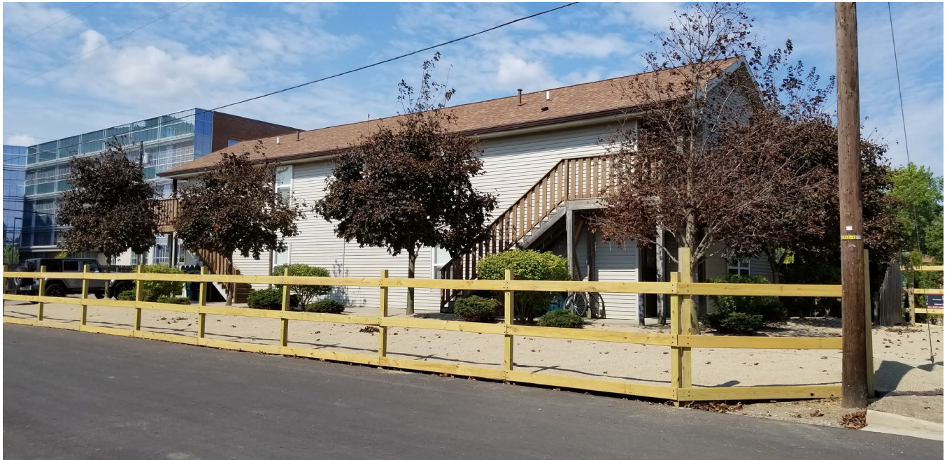
East side of building facing Dicks Street. Apt 4 on top, Apt 1 on bottom.
