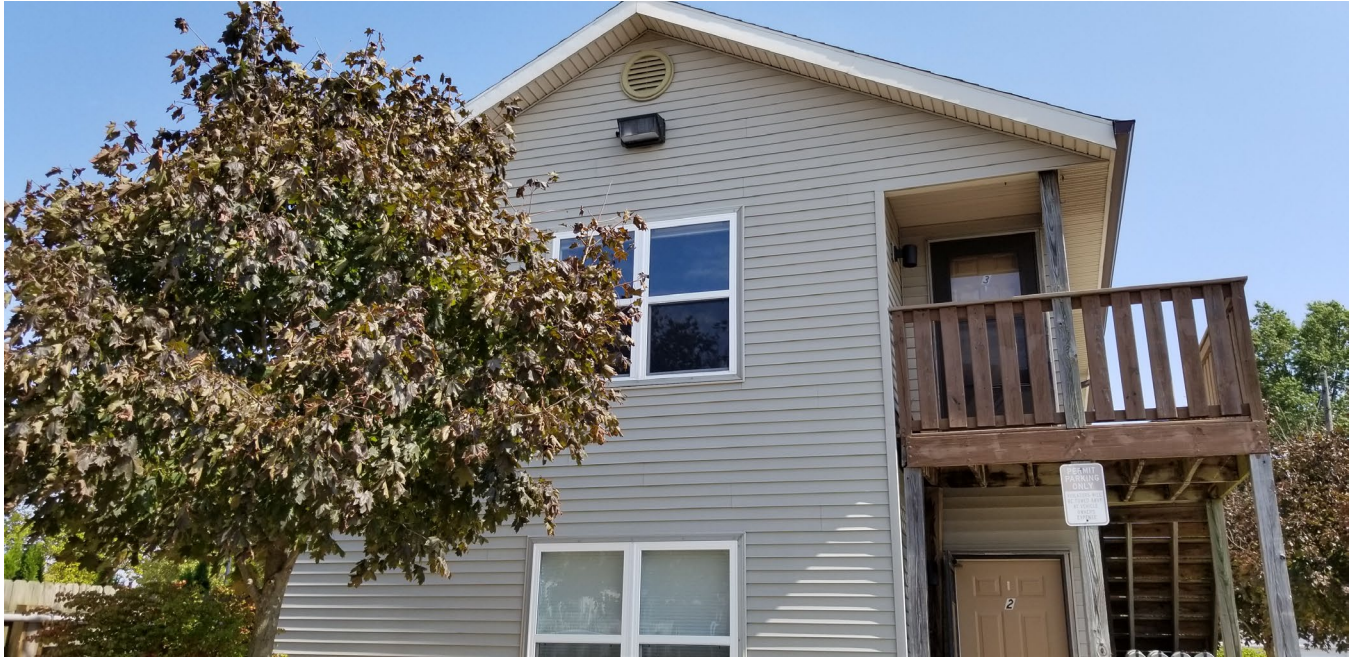
Building Security Lighting-New Stairwells & New Paving 2013.
