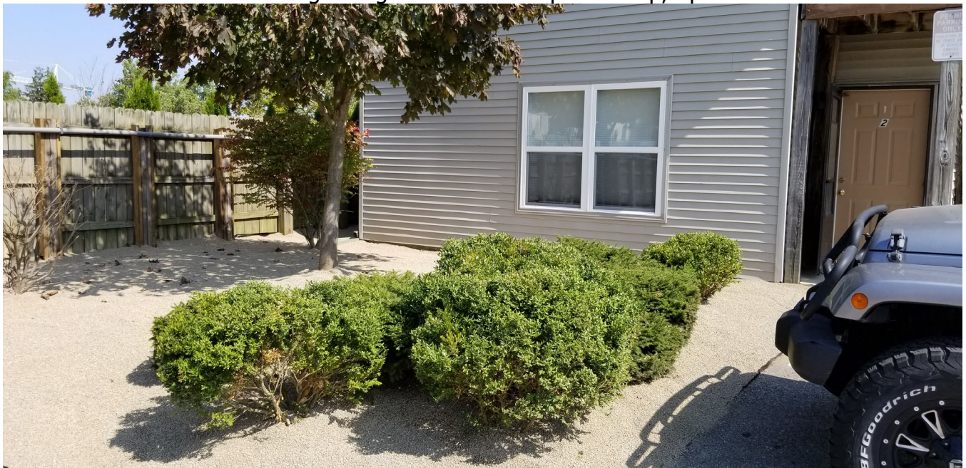
West side of building facing Beechwood parking lot. Apt 3 on top, Apt 2 on bottom.
