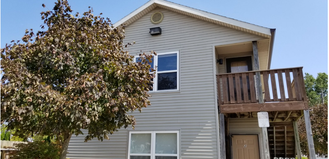
Building Security Lighting-New Stairwells & New Paving 2013.
