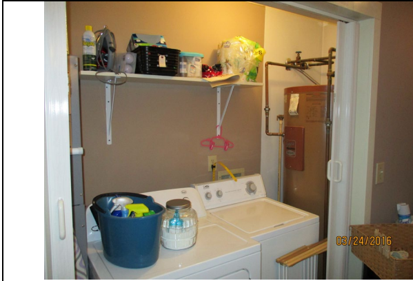
Laundry Area (off Bathroom)
